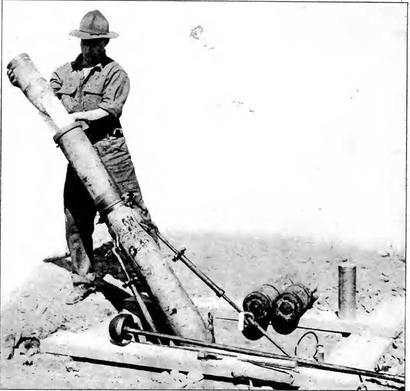
METHOD OF LOADING TRENCH MORTAR.
